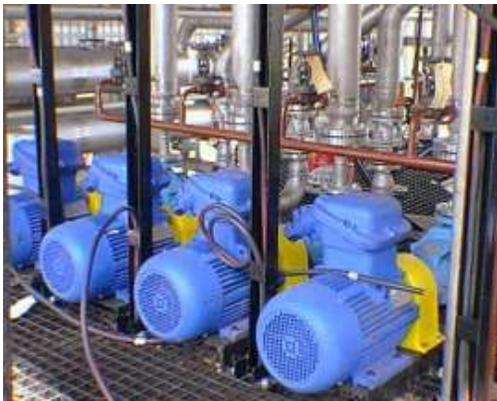
**Figure 1: Some motors operating in hazardous areas do not have IA certification**
